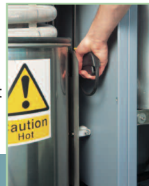
Quick-release tank mechanism
